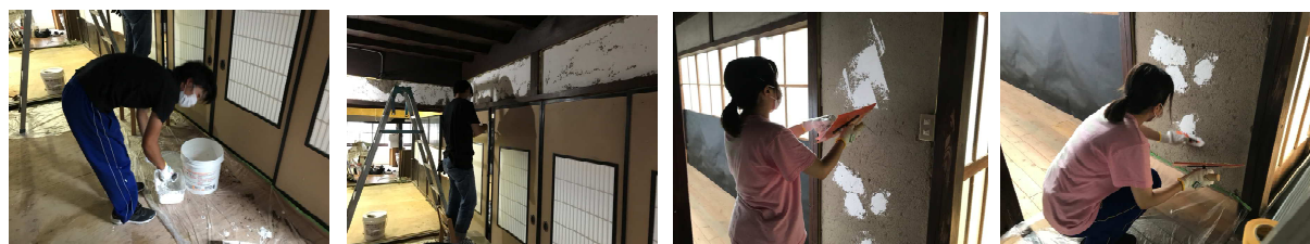
Figure 5 漆喰壁塗り工事
