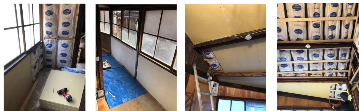
Figure 7 断熱工事
